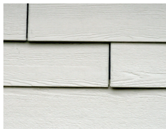
Gaps in Fiber Cement
